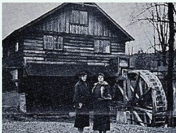
The Mill Built by Jim Kirby in 1922.
